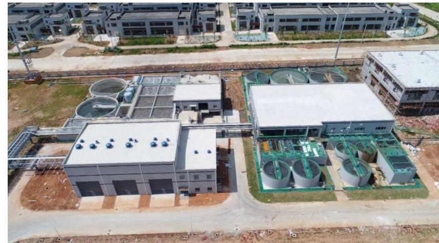
Sewage Treatment Plant + Substation
