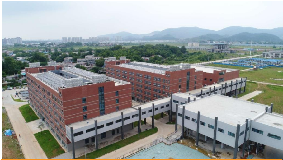
Dormitory + Connecting Bridge over the Factory Area
